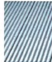
Metal sheet roofing
